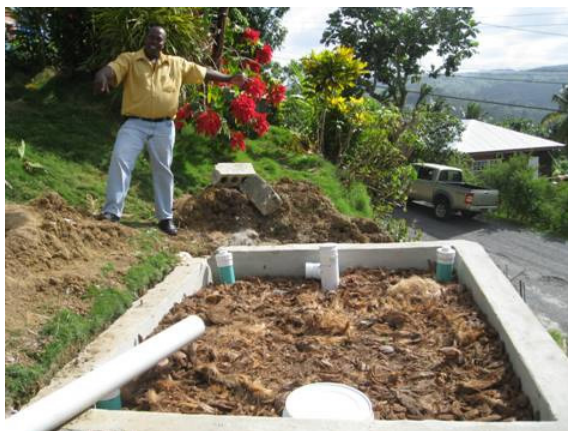
Accessible technology solutions, such as this wetlands filtration system, are being constructed in Saint Lucia as part of an overall approach to managing wastewater in a changing climate. (Photo by Donna Spencer).
