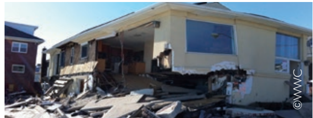
Hurricane Sandy damages.
