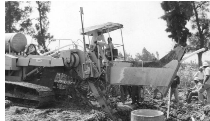
Figure 6. Subsurface drainage system installation
