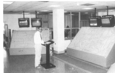
Figure 10. Main control room for the telemetry system showing the MIMIC Board and the monitors
