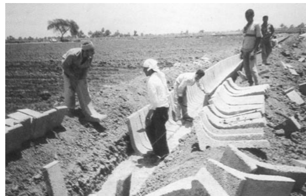
Figure 5. IIP modern gates and new raised mesqa construction
